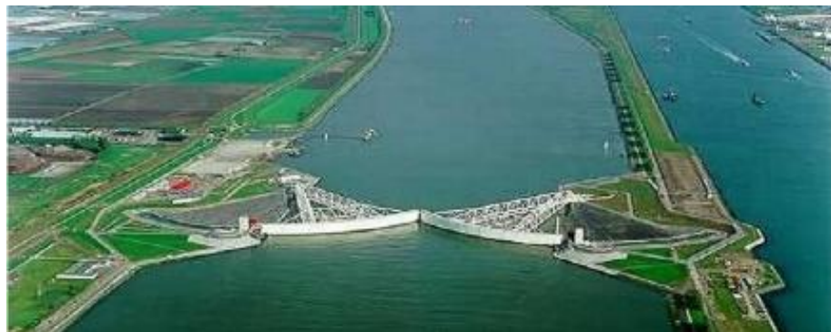
Figure 2: Lock-gate on the "Nieuwe waterweg", Rotterdam (the Netherlands)
